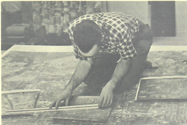
Technician compiles a semi-controlled aerial mosaic. Large county can be covered in a single mosaic.
